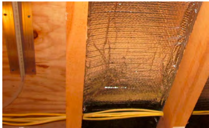
Figure 3-1. Radiant floor heating piping and insulation for the main floor at PB site
