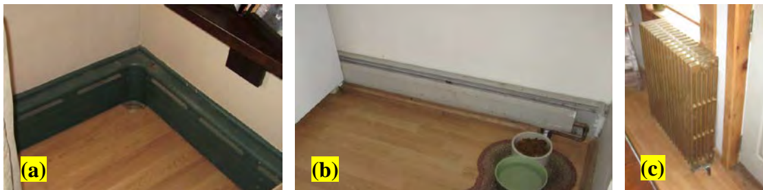
Figure 3-5. Heat emitters used in WPB residential building: (a) cast iron baseboard (~ 9 m long); (b) fin-tube baseboard (~ 7 m long); (c) cast iron radiators
