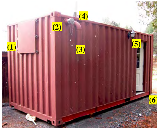
Figure 3-2. Parishville boiler (PB) heating system inside an insulated shipping container.
