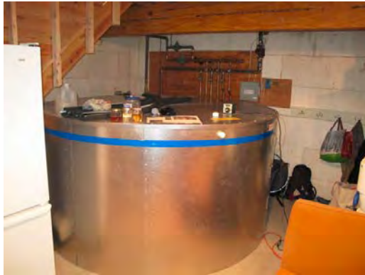
Figure 2-11. Photo of on-site installation (left) and schematic (right) of a typical unpressurized (or open) TES tank flow direction (source: NYSERDA renewable heat NY hydronics training)
